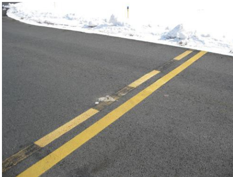
Fig. 6 Non-Movement Area Boundary Marking
